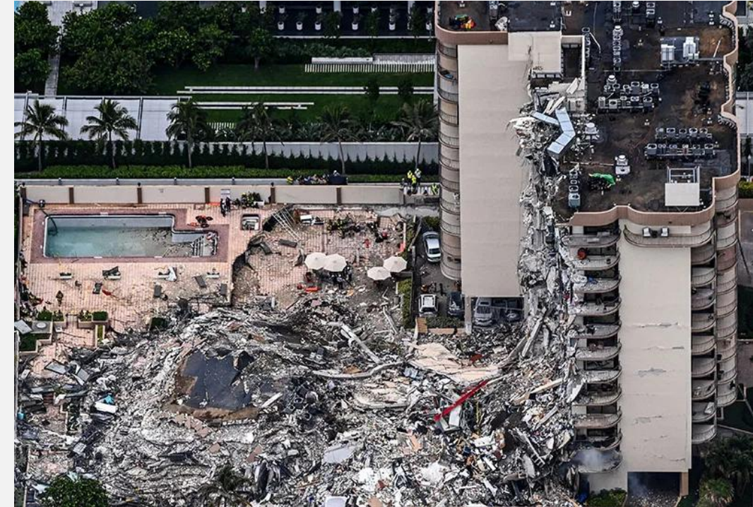
Champlain Towers South– Surfside, Florida
