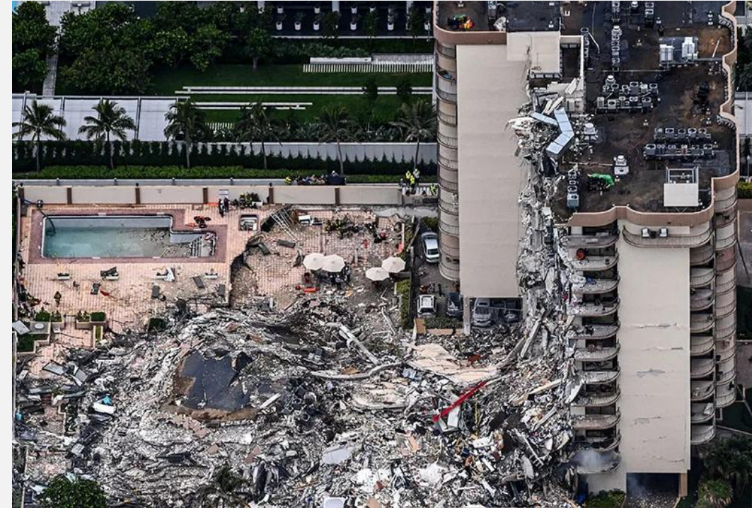
Champlain Towers South– Surfside, Florida
