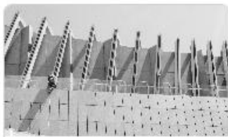
EK Retrofit - Challenges to leasehold retrofit
