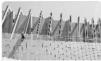
Principles of Maintenance - Chimneys
