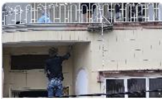
Planning for Maintenance - External Envelope
